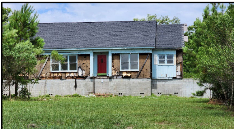
Figure 8: A house in Radium Springs, raised to stave off future floodwaters, is now abandoned. Its future is uncertain. (Photograph courtesy of Denise Clarke-Dumas via the HEAL photovoice process.)
