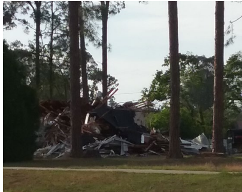
Damage from the windstorms and tornado of 2017.
