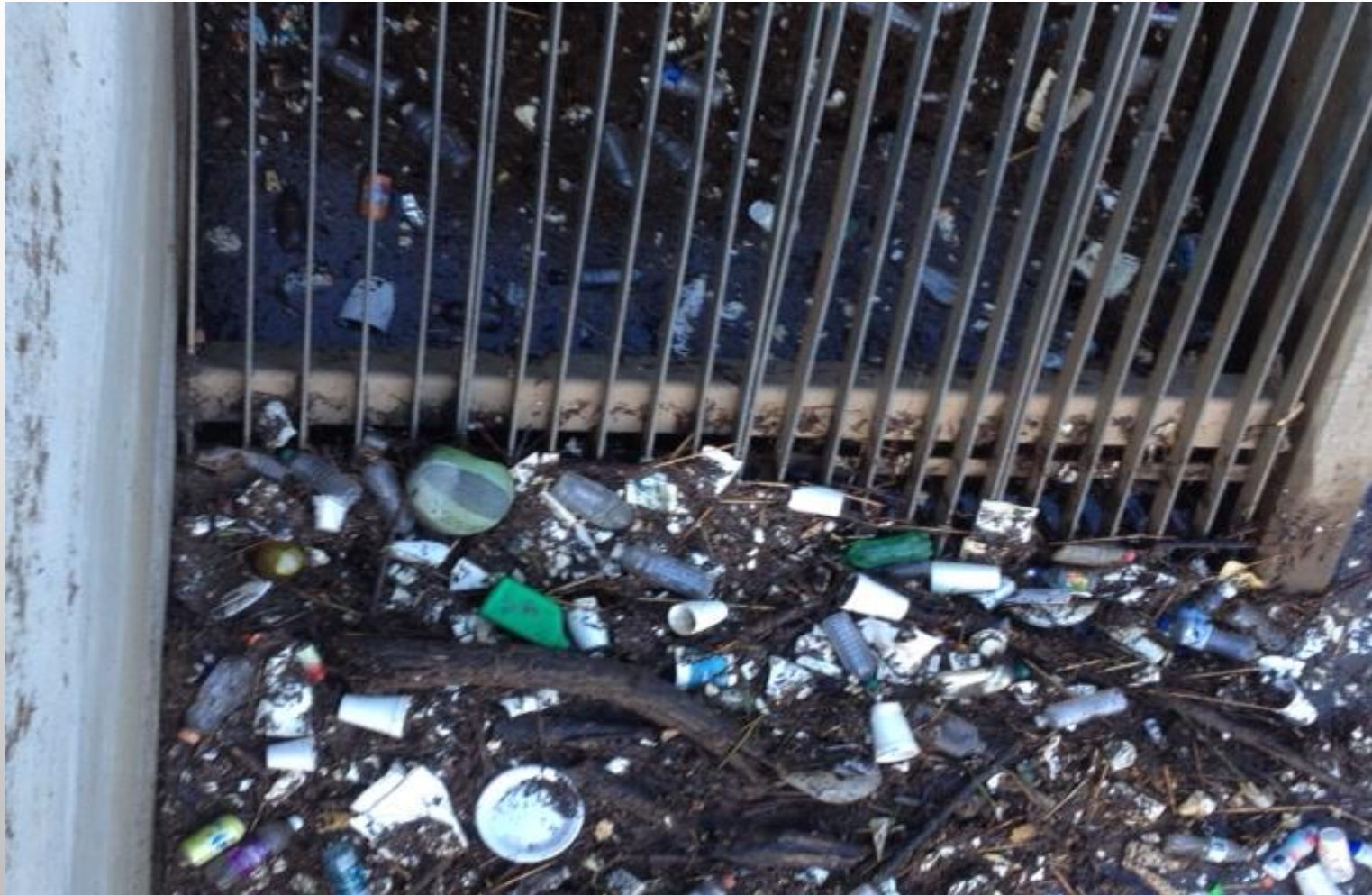
Screens cleaned at Storm Station #103
