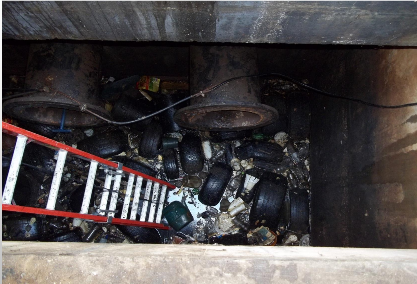
Tire Removal at Storm Station #76
