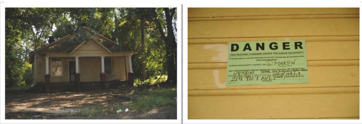
Figure 11. This house, on W. Tift Avenue between Washington and Jackson, has been identified as uninhabitable due to unsafe plumbing hazards.
