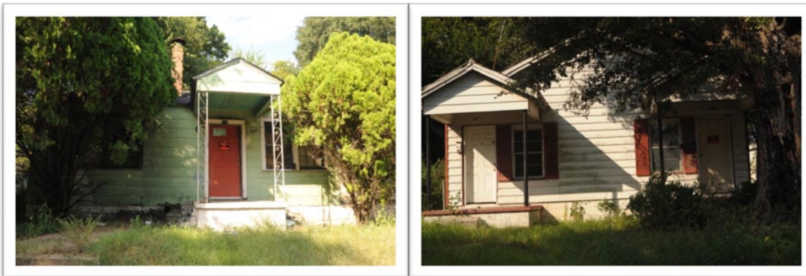
Figure 28. These two homes are located along Byron Road. Byron is a very short road that runs diagonally from Pine Ave to Broad Ave. Most of the homes on this street are vacant and several are deemed unsafe for human occupancy.
