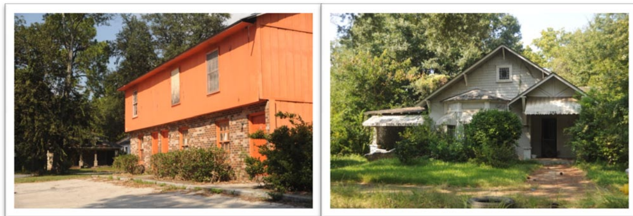
Figure 8. These two dwellings are located on 1 st Avenue between Washington and Jackson. The apartment building on the left is vacant with some boarded up windows and is need of some repairs. The house in the picture on the right is vacant with a couch in the driveway and an old, used tire in the front yard. The shrubs are overgrown with vines growing on the house.
