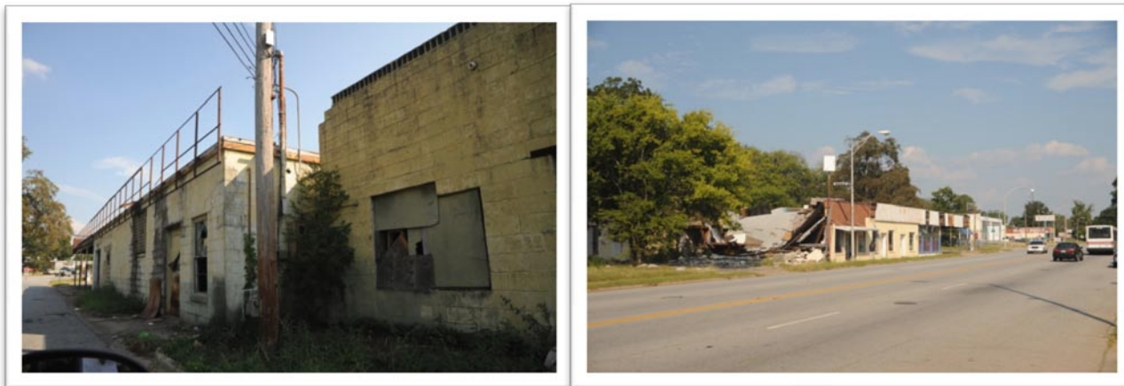
Figure 15. The picture on the left is of the rear of the vacant business at 731 W. Broad Ave. The photo on the right shows the front of the building along Broad Ave. The roof is caved in on the west side of the property.
