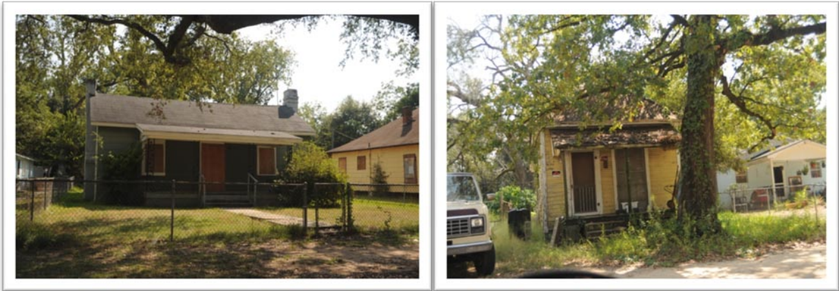
Figure 4. These homes are located on 6 th Avenue, between Washington and Jackson. The windows are boarded up and it appears that they are vacant.
