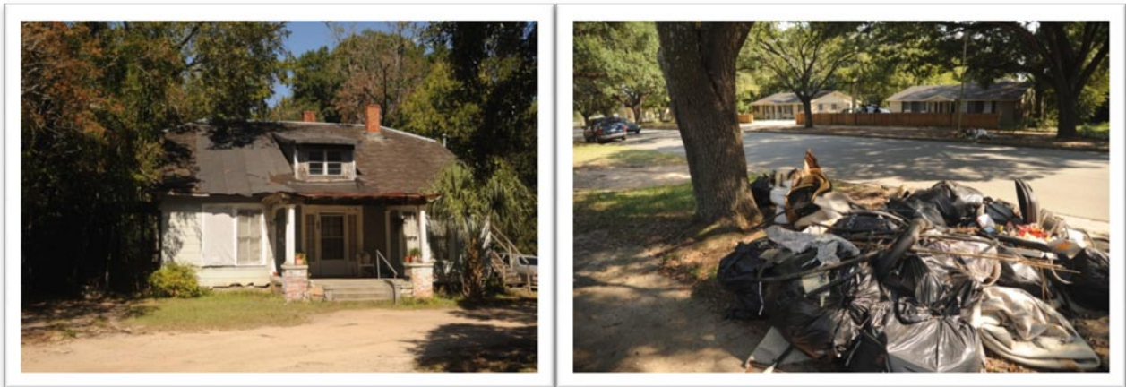
Figure 10. These two pictures are also from W. Society Avenue. The house on the left has some windows boarded up and is in need of roof repairs. The roof, left of the dormer, has no shingles. The photo on the right shows a large pile of trash just off the street and also a smaller pile of trash on the other side of the street.
