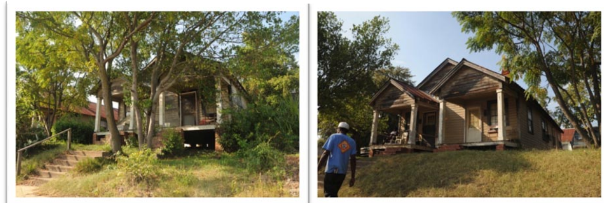
Figure 19. The duplex pictured on the left is 851 W. Broad Ave. Both duplexes are aged and in need of some repairs. They are inhabited, but without being painted, along with other obvious aesthetic needs, their appearance adds to the blight found on W. Broad Ave between downtown and Slappey Blvd.
