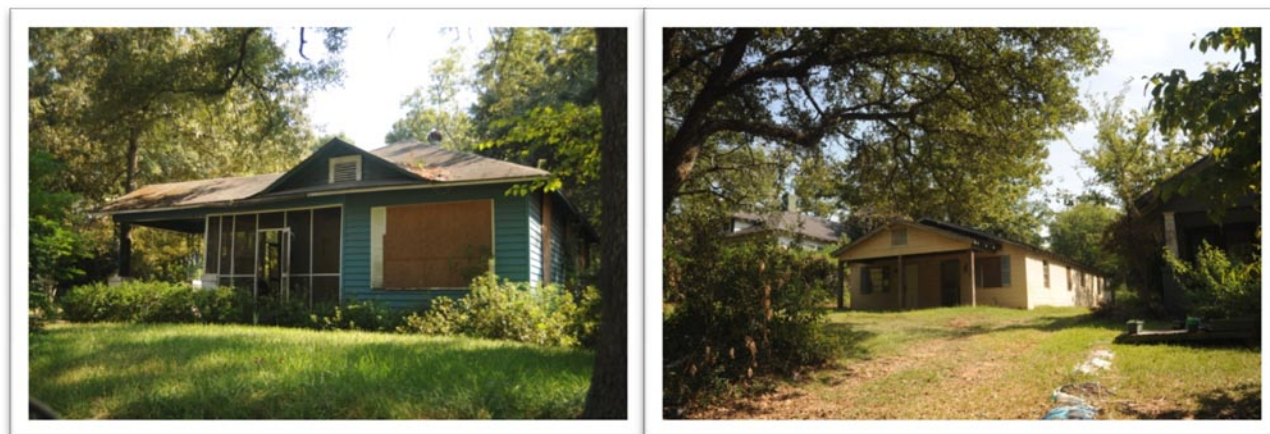
Figure 7. These homes are located on 2 nd Avenue, between Washington and Jackson. The windows are boarded up and they appear to be vacant.
