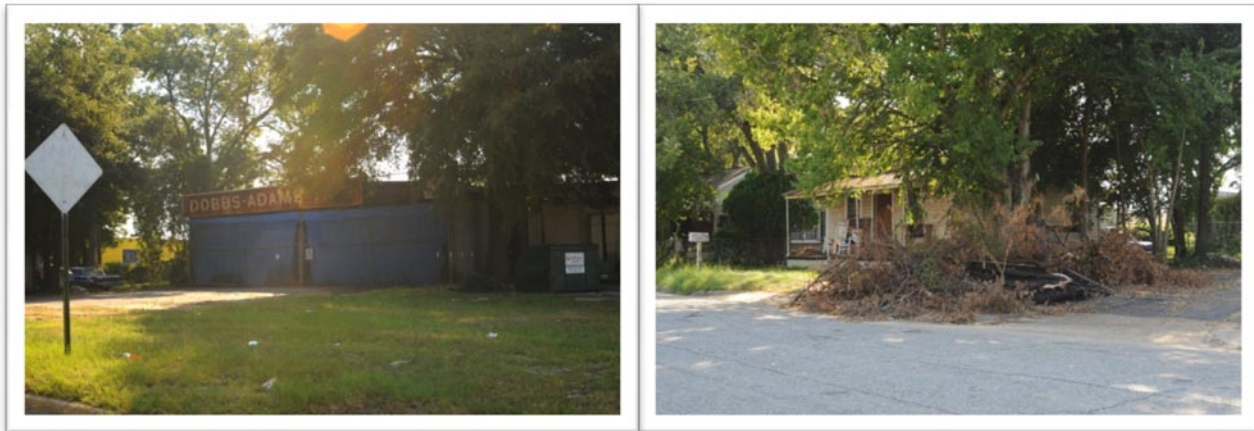
Figure 25. These two properties are located along Haley Street, north of Broad.
