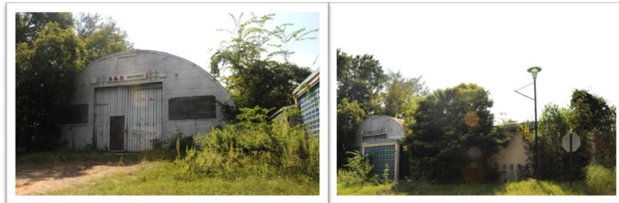
Figure 1. These two buildings are located along Lipsey Dr, which is part of the Roosevelt corridor. The building on the left is covered with profanity-laden graffiti and the building on the right is almost totally covered in vines and overgrown shrubs and trees.
