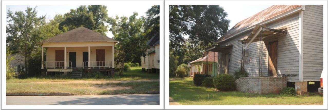
Figure 9. These two dwellings are located on W. Society Avenue between Washington and Jackson. The duplex on the left is boarded up and appears to be vacant. The duplex on the right is also boarded up and in need of significant repairs.
