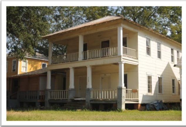
Figure 12. This apartment building on W. Tift has some windows boarded up and appears to be vacant. It is attached to another property in need of repairs that runs along Washington Street.
