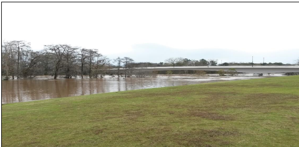
Broad Avenue Bridge January 2016
