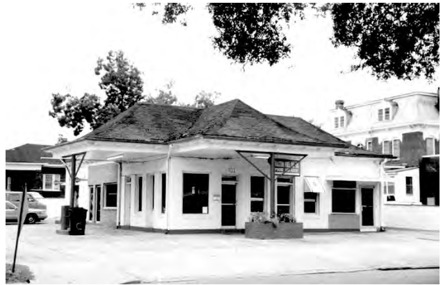
Projecting canopies and large display windows are distinctive features of this early twentieth century gas station.
