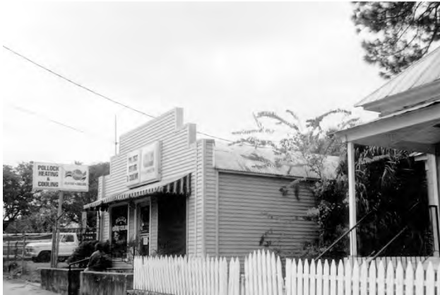
✓ This small commercial building features a barrel-vaulted metal roof with a front parapet wall.
