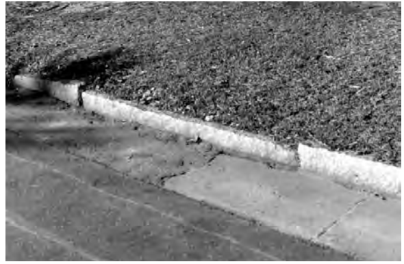
Historic granite curbs
