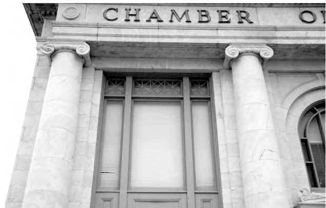
✓ Triple window with diamond-paned transoms.
