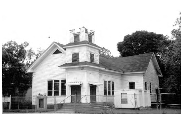
This vernacular frame church on the corner of Washington and Whitney Streets retains its original weatherboard siding and part of its corner tower.
