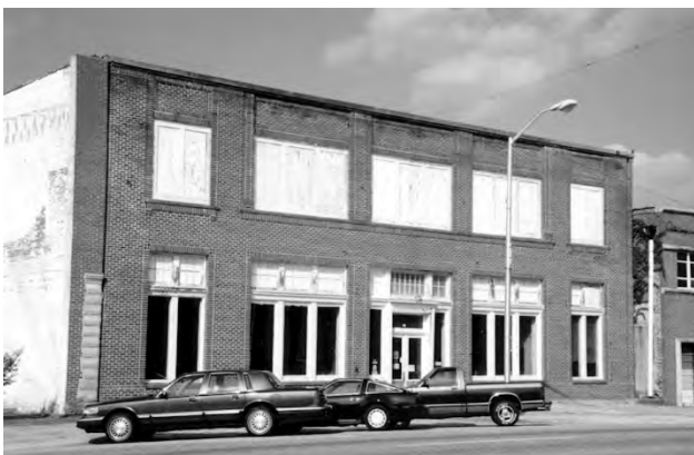
✓ The wood-framed windows and transoms of this lower floor space are intact.
