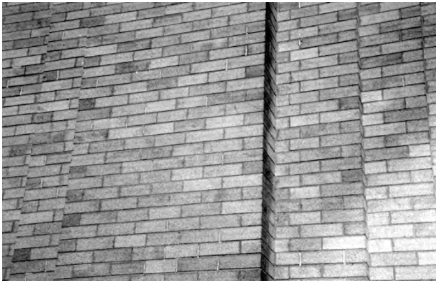
✓ Detail of yellow-brick veneer.
