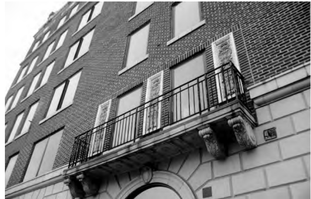
✓ Small balcony with metal balustrade and supported by carved stone brackets.
