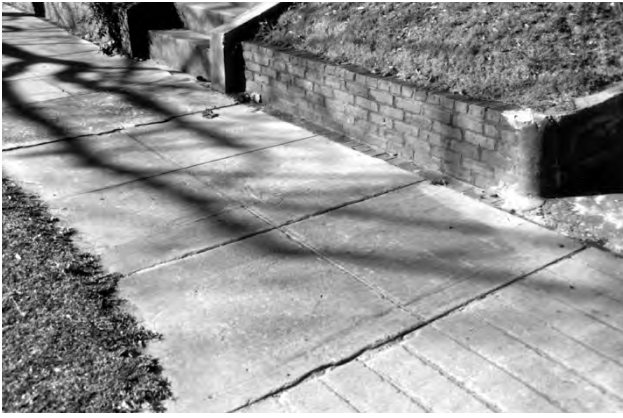
Historic 3' x 3' Albany concrete sidewalk grid.
