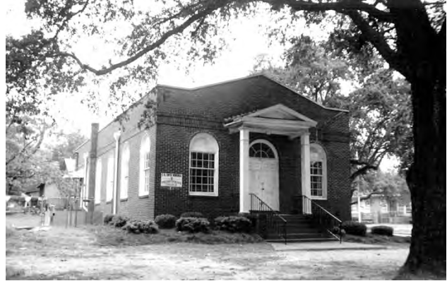
The First Church of Christ Scientist, constructed c1938, features elements of the Neoclassical Revival style.
