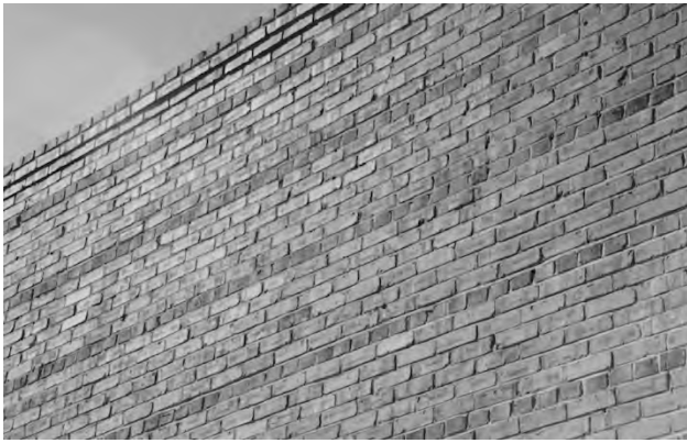
✓ Detail of a common bond brick exterior.
