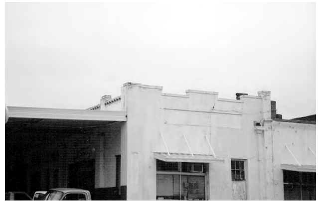
✓ This historic corner gas station and repair shop features a small clay-tile awning on its parapet wall; this clay tile is an important character-defining element of the building and should be preserved.
