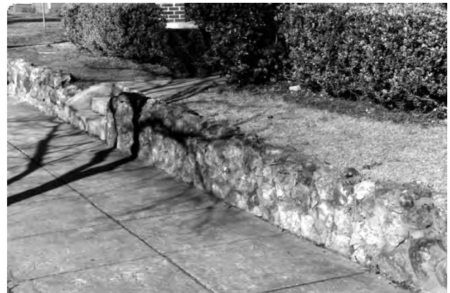
A retaining wall utilizing rough stone.
