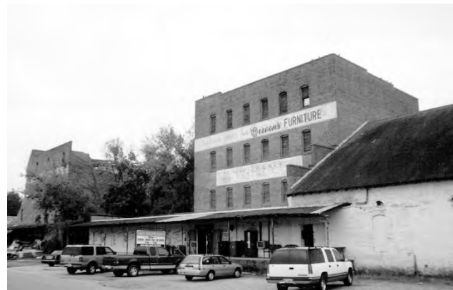
Currently, an antiques business occupies this former manufacturing complex. The exterior loading dock is an important feature of the historic industrial complex that should be retained.
