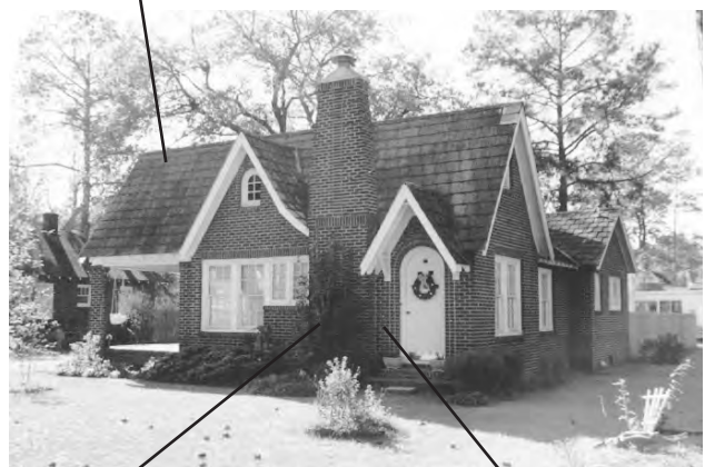
prominent front chimney
