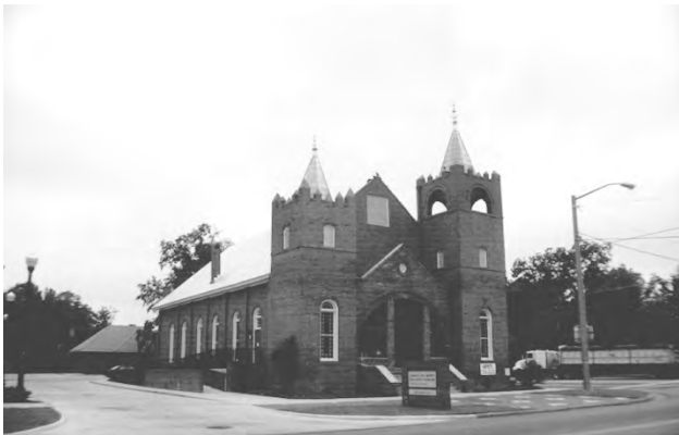
The 1906 Mt. Zion Church features Romanesque Revival-style elements with its prominent brick arched opening and its castellated towers.
