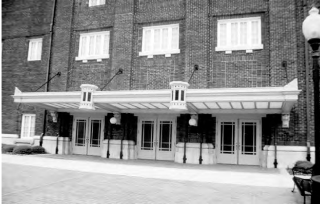
✓ The entrance canopy on the Municipal Auditorium features octagonal, metal light fixtures and scalloped corner decorations.
