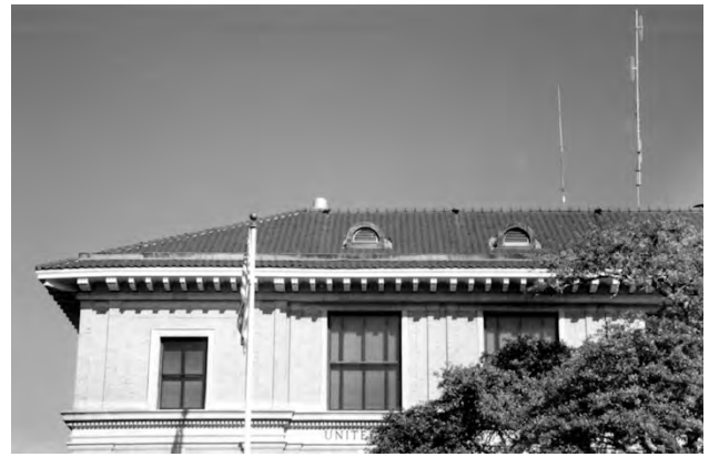
✓ The hipped clay tile roof is a distinctive feature of the U.S. Post Office and Courthouse.
