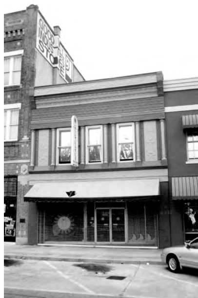
This building is a good example of a two-part commercial block.
