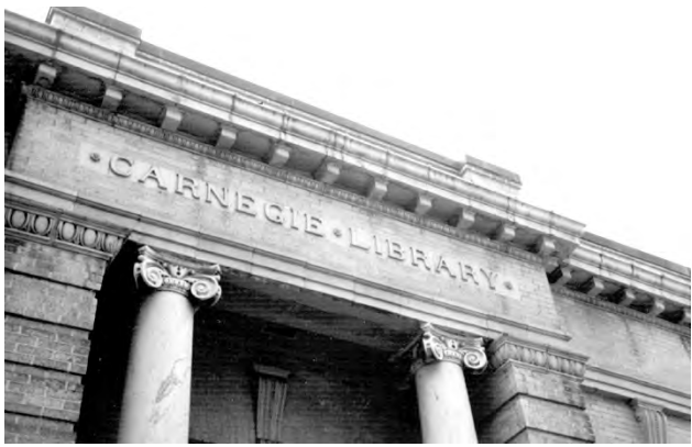
✓ Early twentieth-century classical details of the historic Carnegie Library include Ionic capitals and an entablature.
