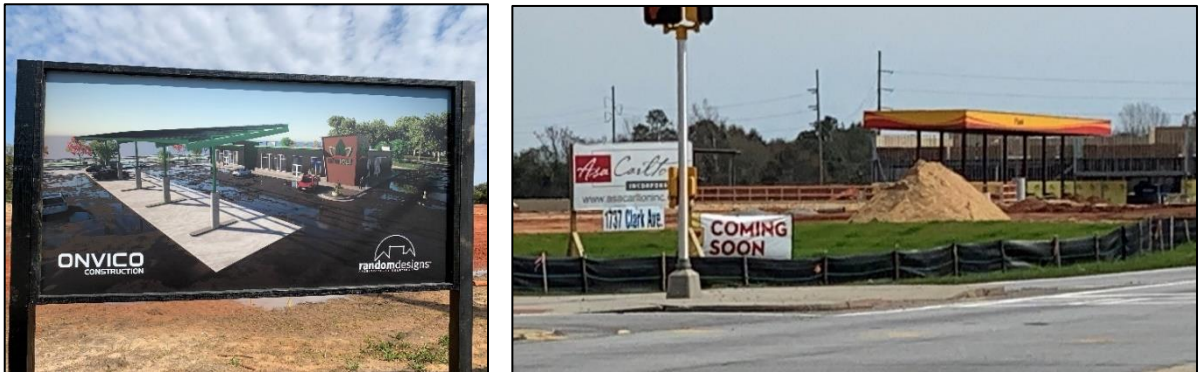
FIGURE 28: NEW COMMERCIAL DEVELOPMENT IS UNDER CONSTRUCTION ON CLARKE AVE AND HIGHWAY 19.
