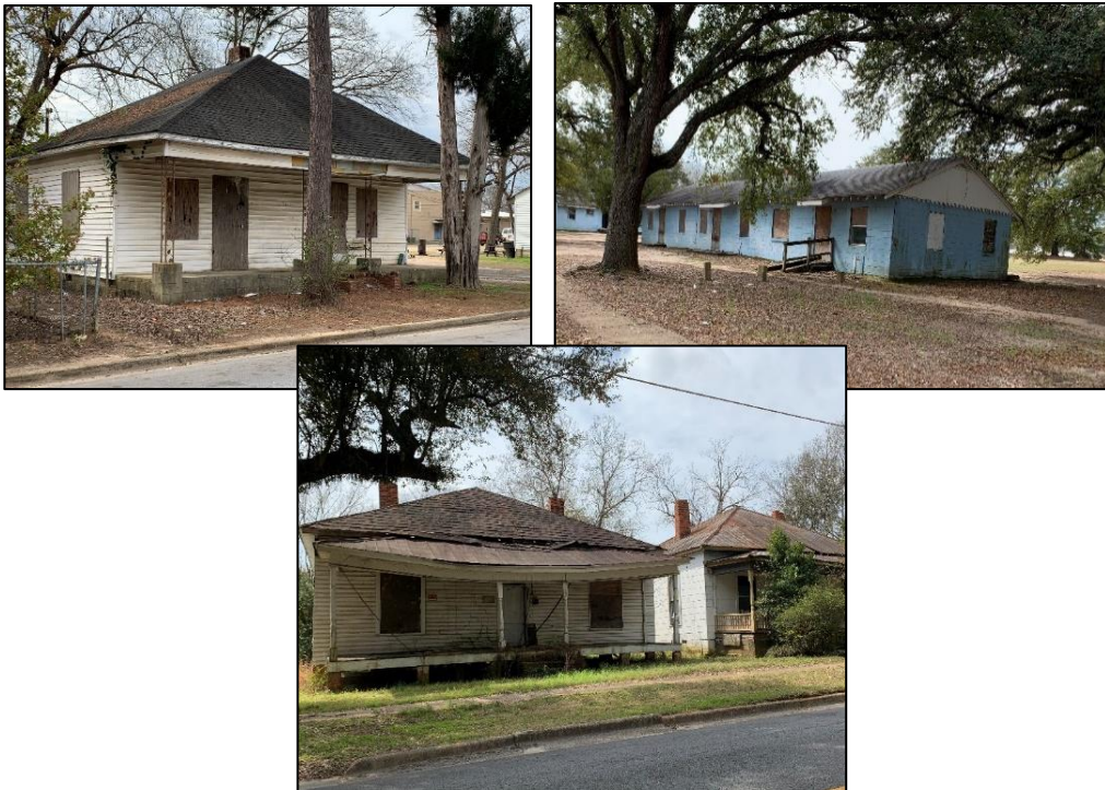
FIGURE 21: VACANT DILAPIDATED HOUSING IS WIDESPREAD IN EAST ALBANY.
